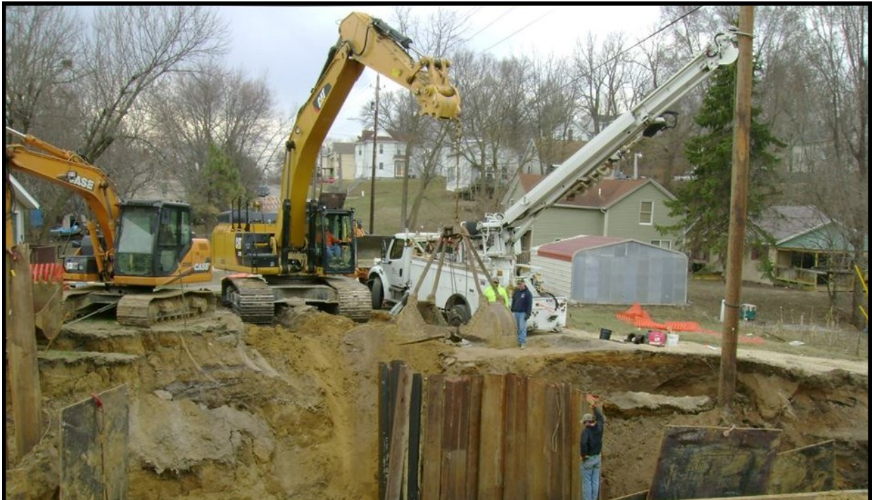
Photo: West Hill Sewer Separation Project
