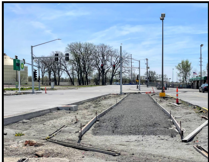
Trail Under Construction Along Warren Street
