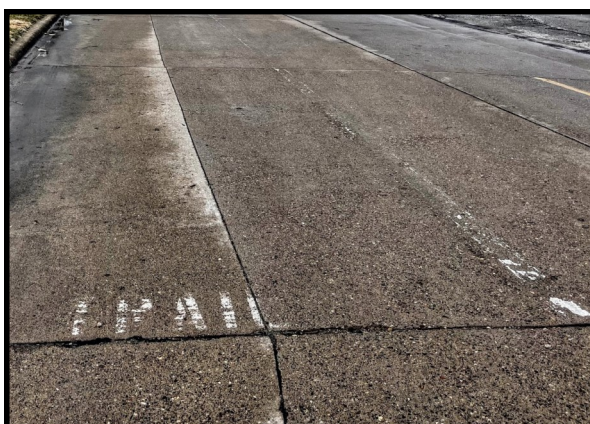
Pavement Marking Delineating the On-street Trail
