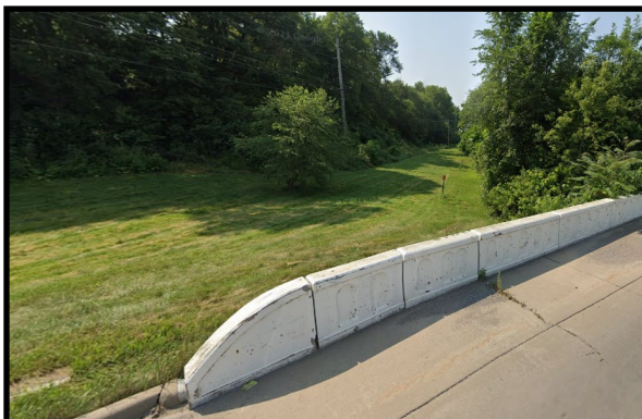
Trail Route Looking South from 5th Street
