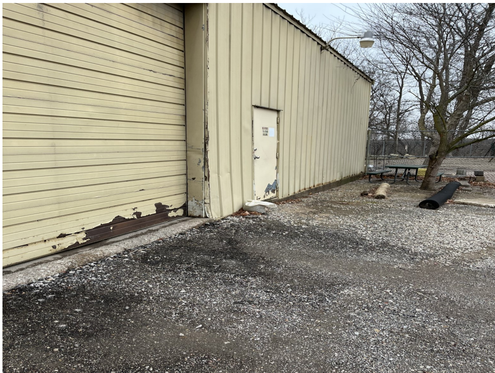
Photo: Current old maintenance building exterior
