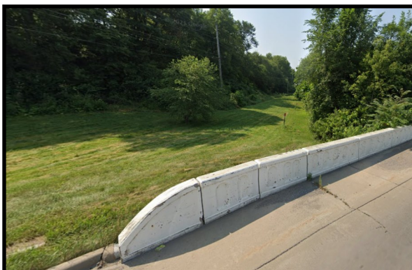
Trail Route Looking South from 5th Street
