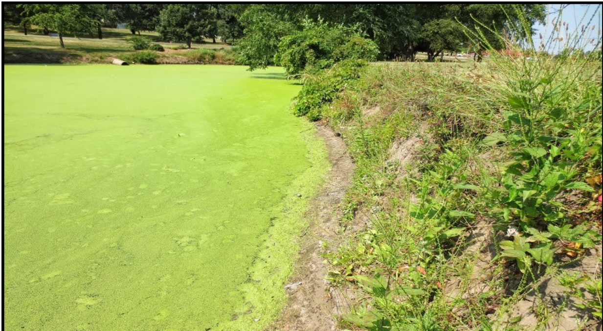
Photo: Erosion at the Weed Park Lagoon
