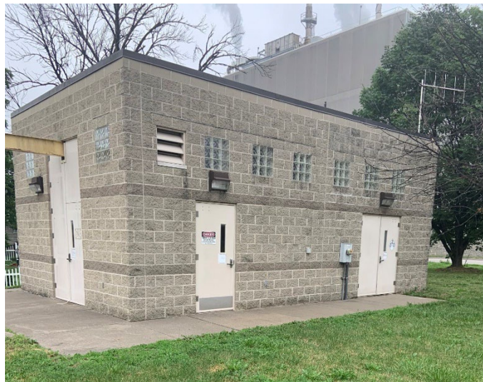
Figure 3-15: Exterior of Miles Lift Station
