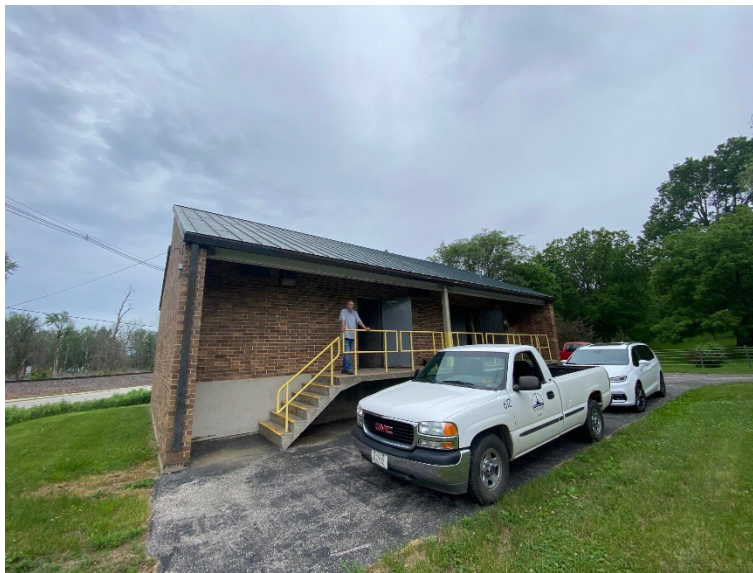
Figure 3-7: Exterior of Canon Lift Station
