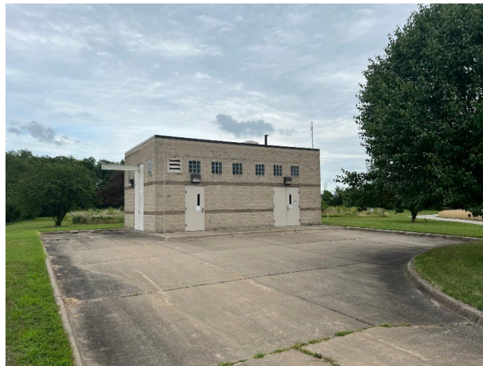
Figure 3-13: Exterior of Sampson Lift Station
