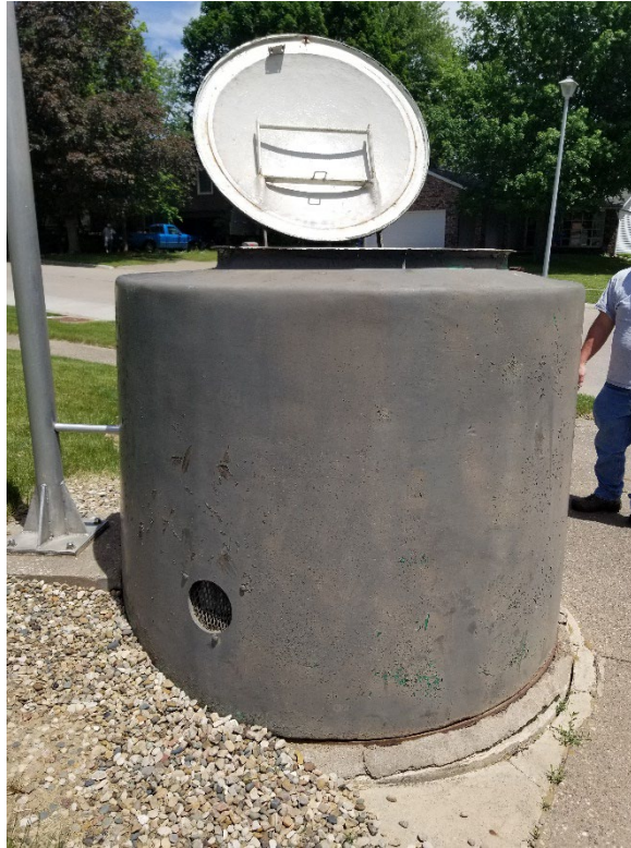
Figure 3-29: Exterior of Tanglefoot Lift Station
