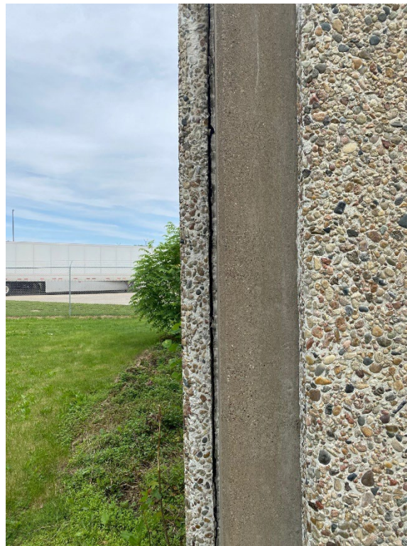
Figure 3-22: Isett Exterior Wall
