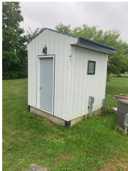
Figure 3-28: Exterior of Sunset Lift Station
