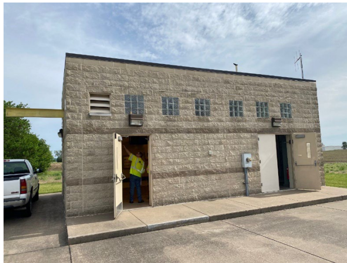
Figure 3-18: Exterior of 57th Street Lift Station
