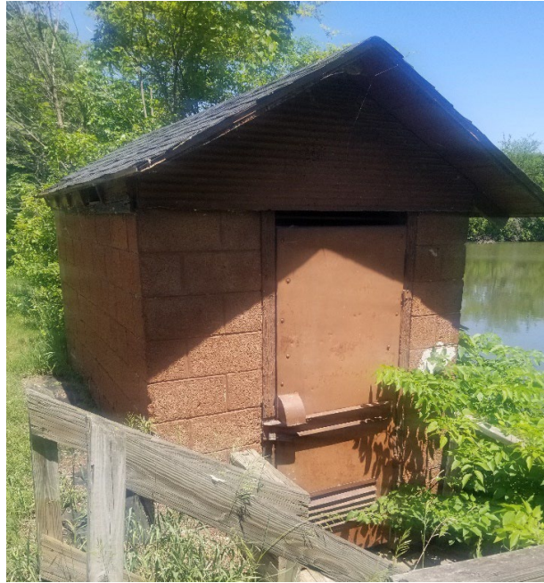
Figure 3-12: Exterior of Slough Lift Station
