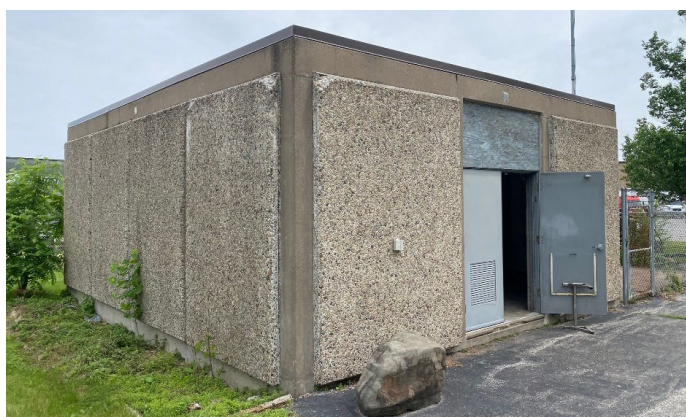
Figure 3-21: Exterior of Isett Lift Station
