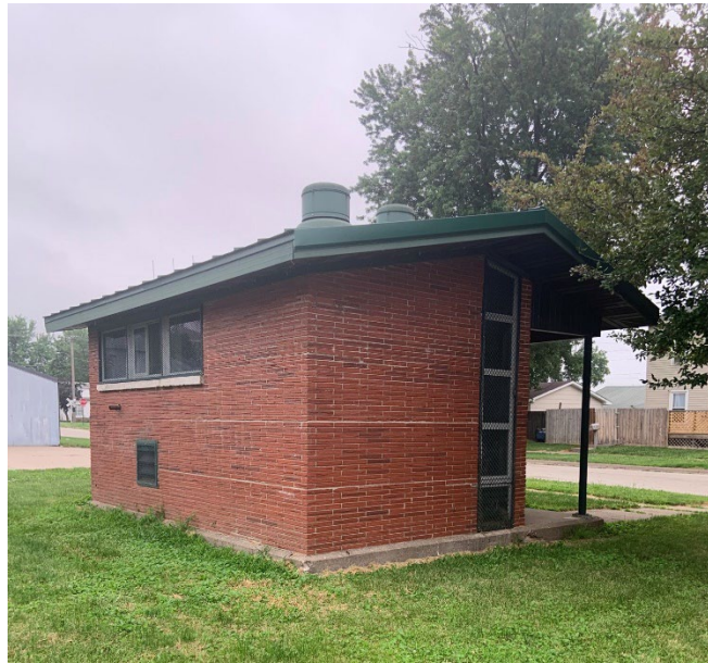
Figure 3-14: Exterior of Schley Lift Station
