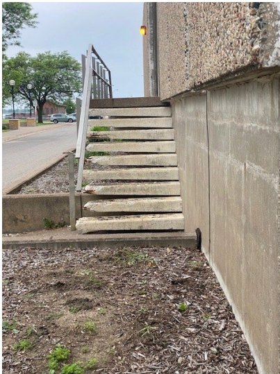
Figure 3-2: Papoose Exterior Stairs
