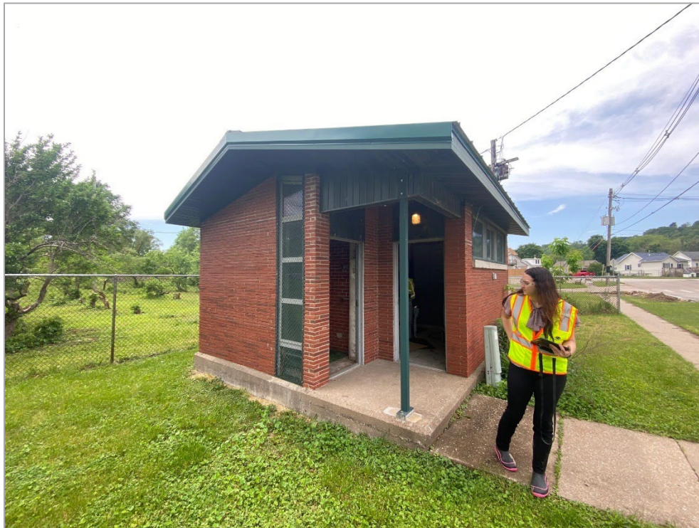
Figure 3-11: Exterior of Bond Lift Station
