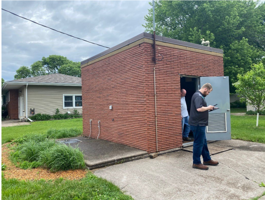
Figure 3-10: Exterior of Houser Lift Station
