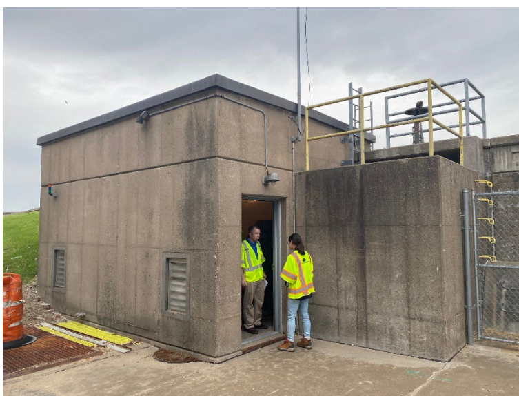
Figure 3-5: Exterior of Stormwater Lift Station
