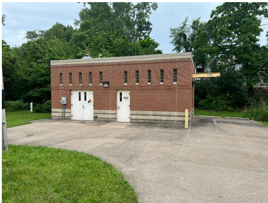
Figure 3-8: Exterior of Tipton Lift Station
