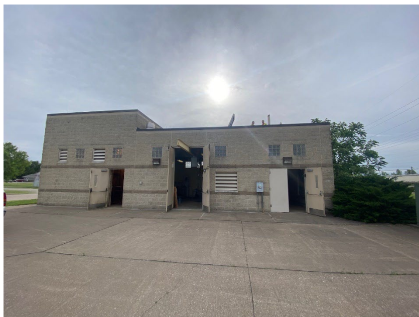
Figure 3-16: Exterior of Stewart Road Lift Station
