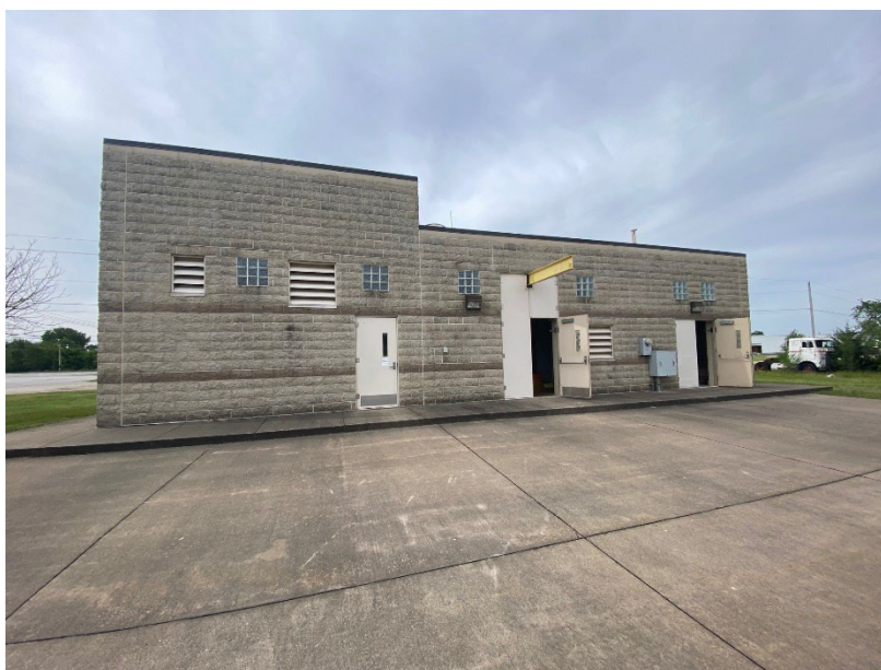
Figure 3-19: Exterior of Progress Park Lift Station
