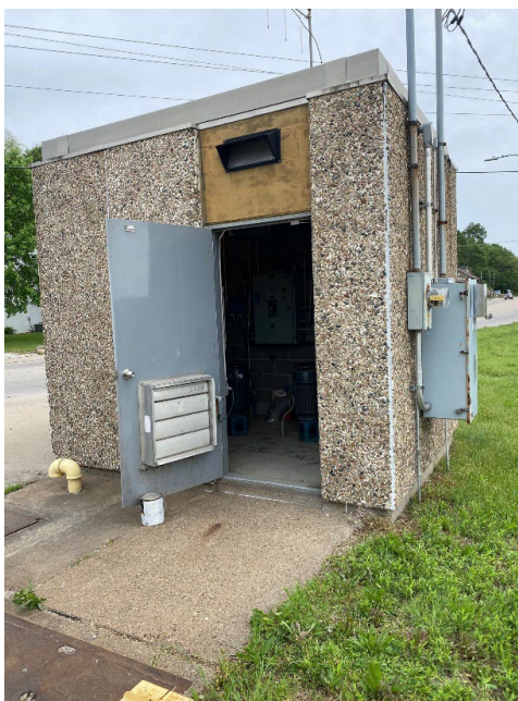
Figure 3-20: Exterior of Hershey Lift Station
