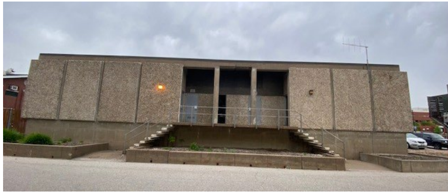
Figure 3-1: Exterior of Papoose Creek Lift Station
