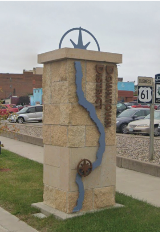
Existing Stone Pillar
