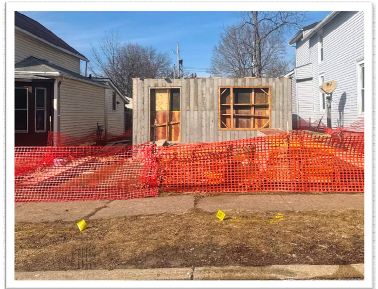
New Home Under Construction at 409 E. 6 th Street
