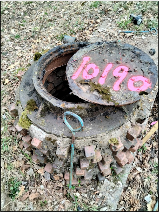
PHOTO 2: MANHOLE 5455 BRICK RISER SECTIONS ON UWBS
