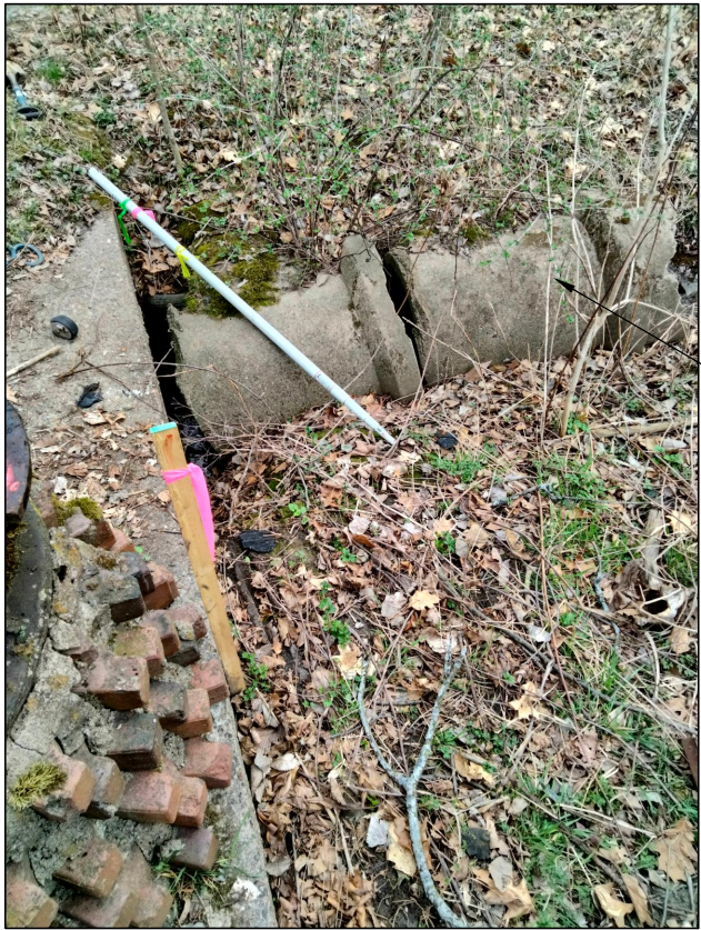
PHOTO 1: UWBS BROKEN PIPE SOUTHEAST OF UWBS
