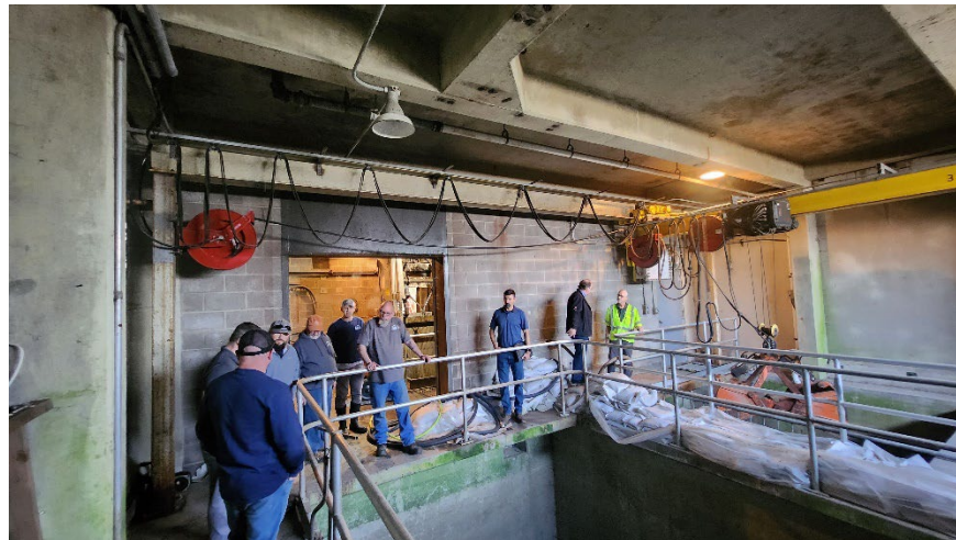
Figure 2-8: Diversion Chamber Room
