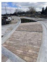
4 SECTION: PAVERS / 6" SLOPED CURB SCALE: 1"=1'-0"
