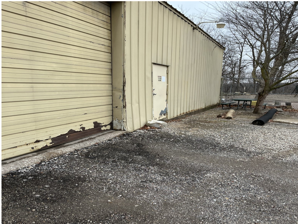
Photo: Current old maintenance building exterior
