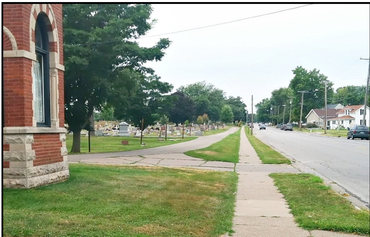
Photo: Proposed Project Area for Barrier Fence
