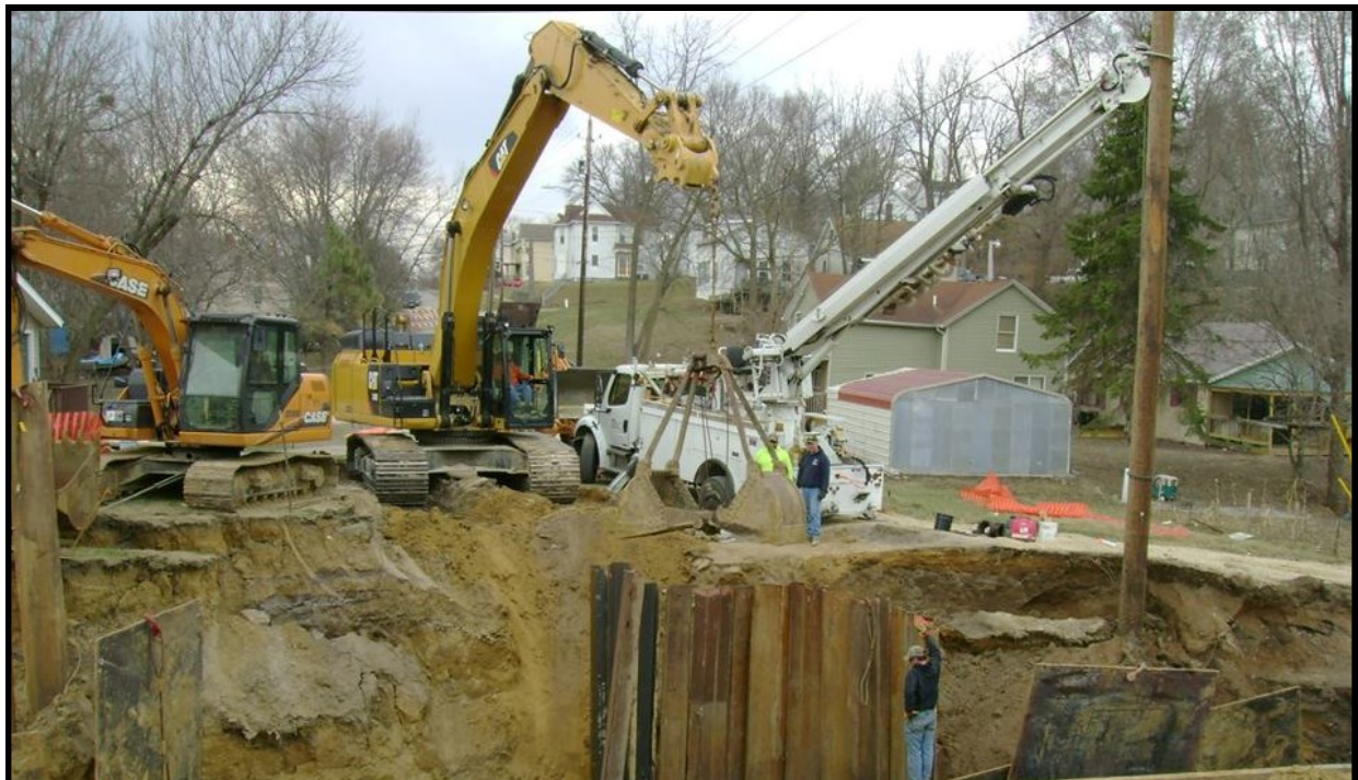
Photo: West Hill Sewer Separation Project
