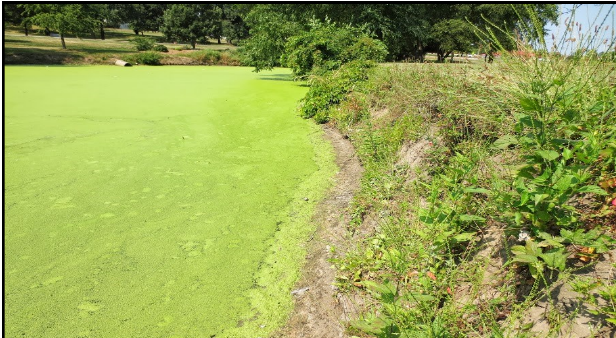
Photo: Erosion at the Weed Park Lagoon
