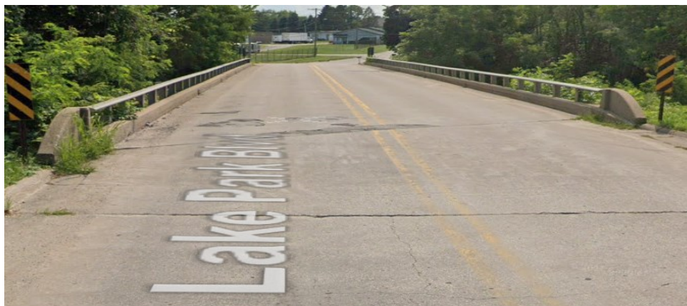
Project Location—Lake Park Blvd Bridge
